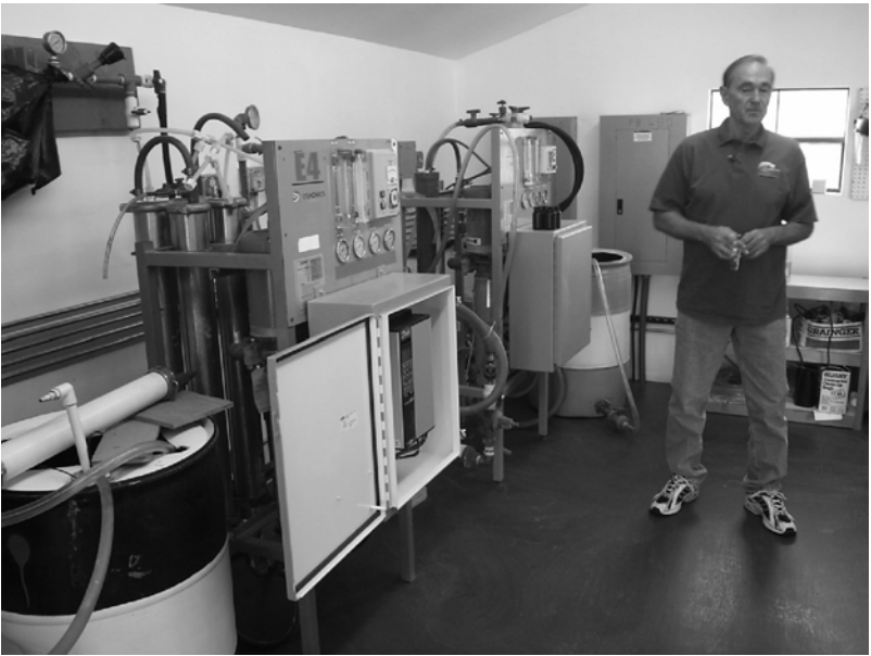
Photo 2. Dr. Tarquin standing in front of Pilot Nanofiltration and RO Membranes (Photograph by Michael Fahy 2006, with permission from El Paso Water Utilities, El Paso, TX)
