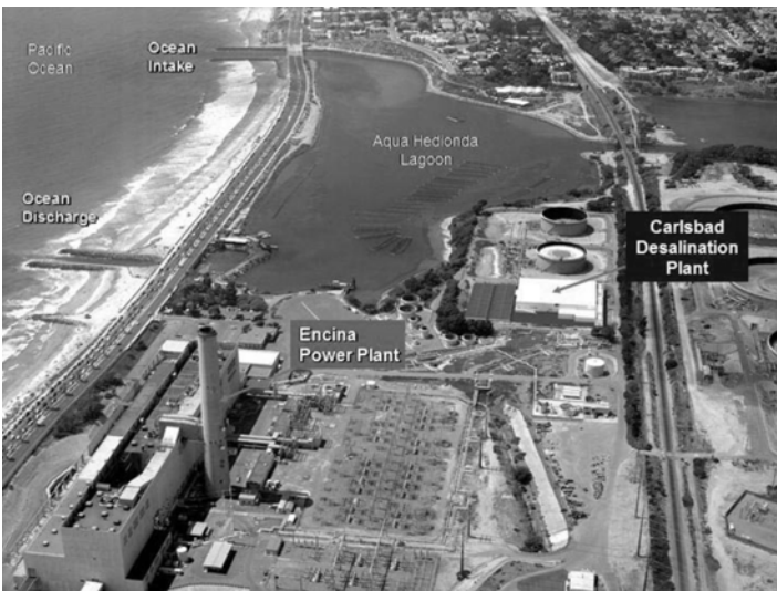
Figure 2. Carlsbad Seawater Desalination Project (Photograph by Nikolay Voutchkov 2004, with permission from Water & Wastewater.com)
