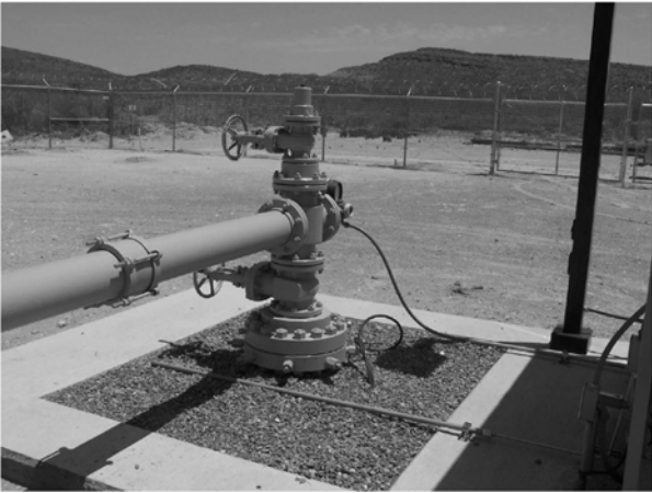
Figure 2. Well-head (Photograph by Eric Bangs 2007, with permission from El Paso Water Utilities, El Paso, TX)
