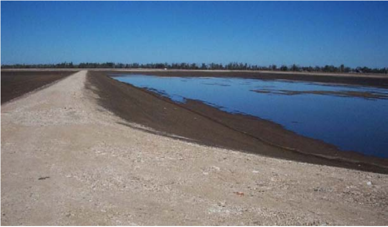
Figure 2. Lined evaporation ponds (Dalby Regional Council Drought Management Plan 2009, with permission from Western Downs Regional Council, formerly Dalby Town Council).
